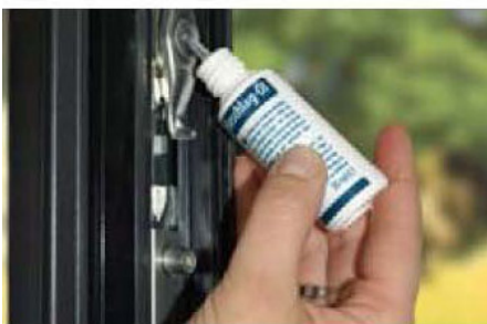
Maintenance of the fittings
