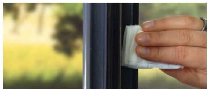
Maintenance of the gaskets
