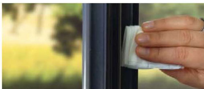
Maintenance of the gaskets
